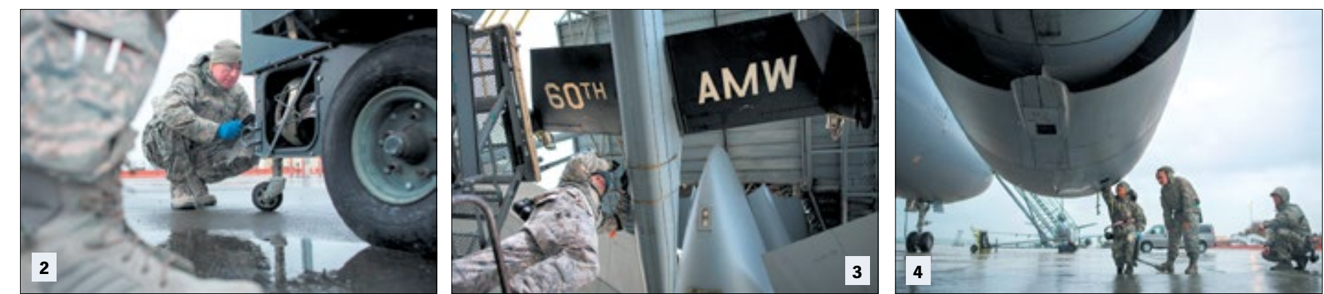
2) Staff Sgt. Steve Perron, 349th Aerospace Generation Equipment Flight mechanic, inspects an engine-driven generator Feb. 6 at Travis Air Force Base, Calif. Because generators can remain stationary and unused for significant periods of time, they must be periodically inspected to guard against low batteries, low tire pressure and fuel issues before they are delivered to aircraft mechanics on the flightline. 3) Staff Sgt. Charles Womack, 349th Maintenance Squadron crew chief, replaces a panel on the boom of a KC-10 Extender Feb. 7 at Travis Air Force Base, Calif. 4) Tech. Sgt. Benjamin Perdido, Staff Sgt. Derrick Miller and Tech. Sgt. A.J. Hunt, 749th Aircraft Maintenance Squadron crew chiefs, conduct an operations check on the engine of a KC-10 Extender Feb. 9 at Travis Air Force Base, Calif.
